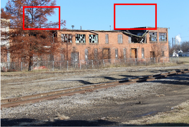
Photo 1 – Area-A South Wall
