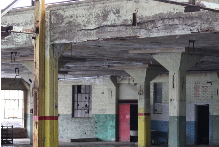
Photo 18 Interior of Areas-D
