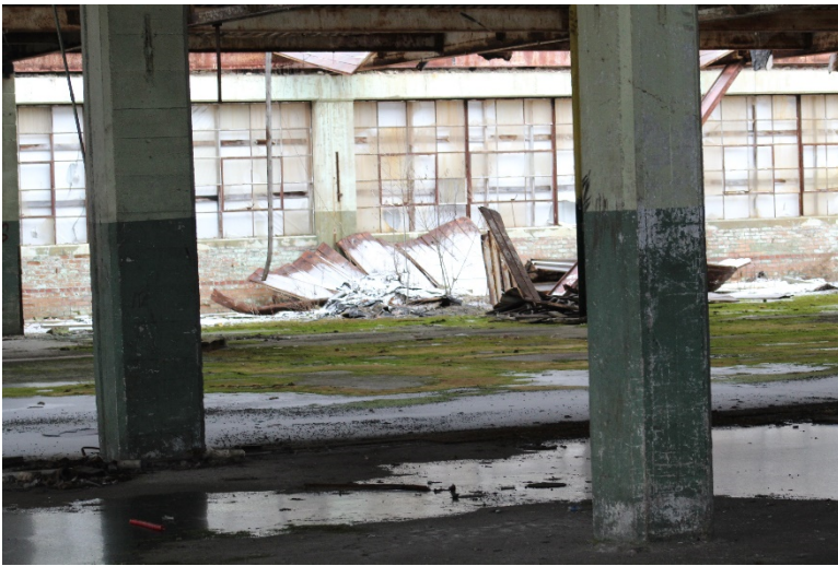
Photo 14 Interior of Area-C & D
