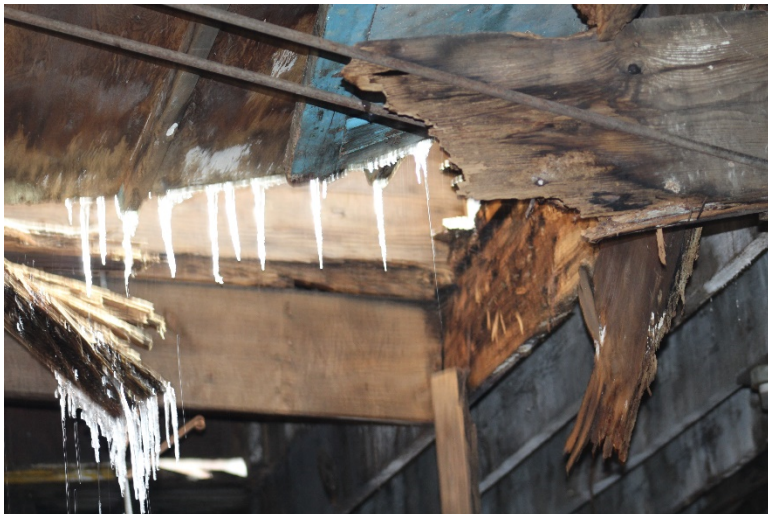
Photo 4 Area-A Roof Section
