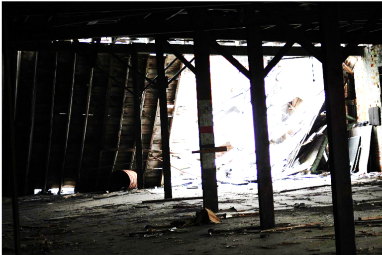
Photo 5 Area-A Roof Collapse
