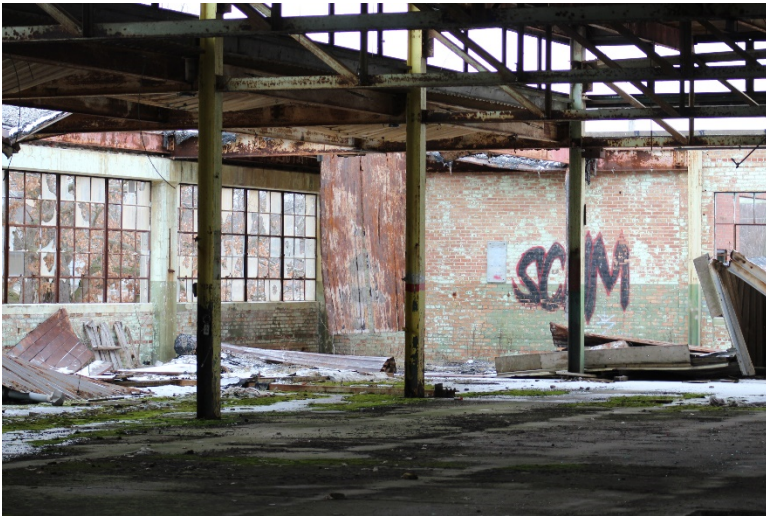
Photo 13 Interior of Area-C
