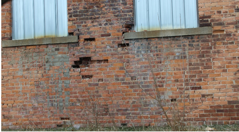
Photo 6 Area-A East Wall Brick Work
