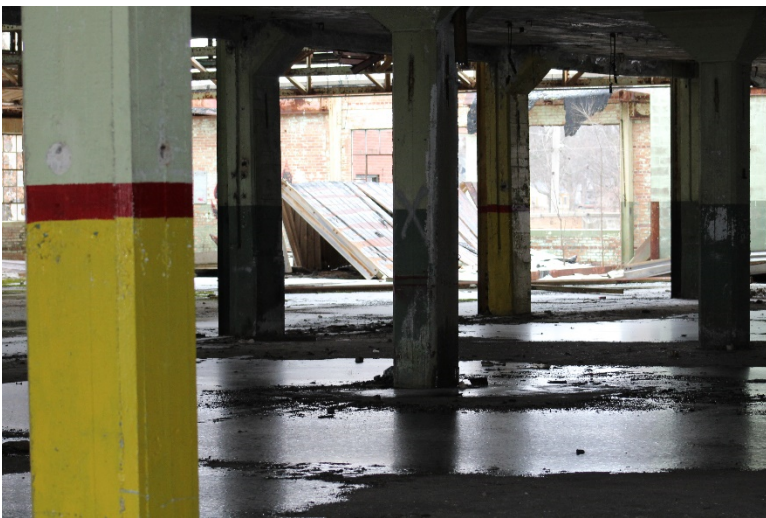
Photo 15 Interior of Area-C
