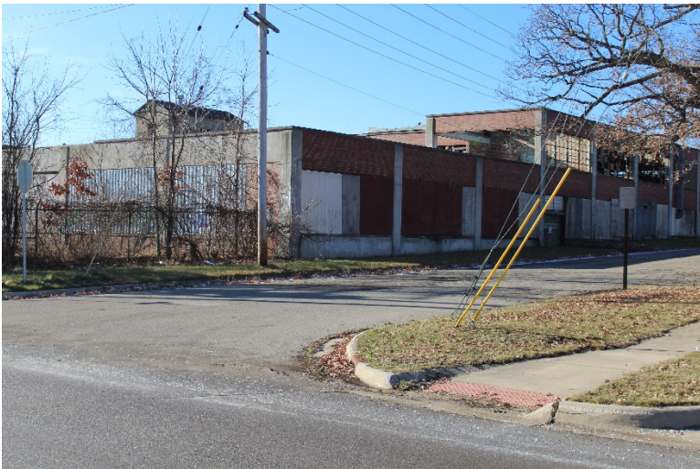
Photo 10 Exterior North Wall Area-C
