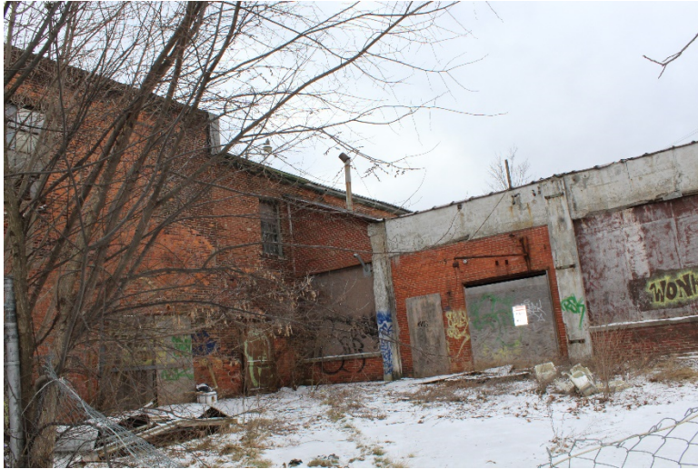
Photo 7 Area-B East Wall
