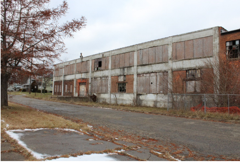
Photo 25 South Wall Area-D
