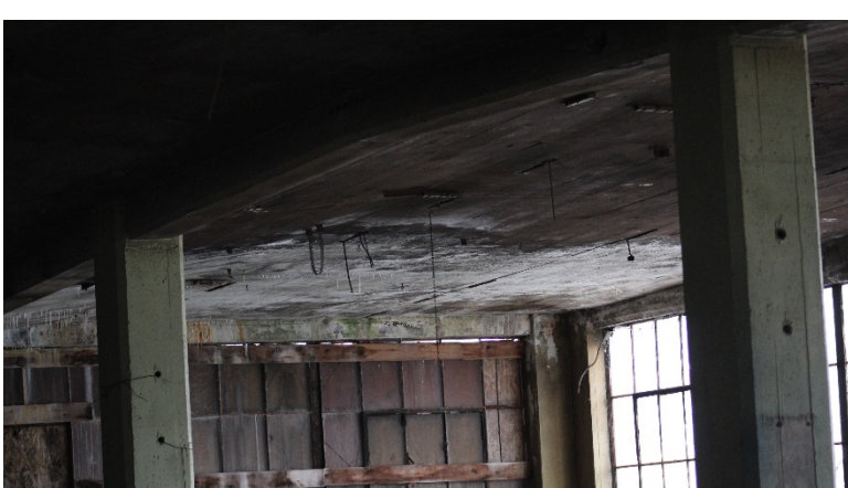
Photo 17 Interior of Area-D
