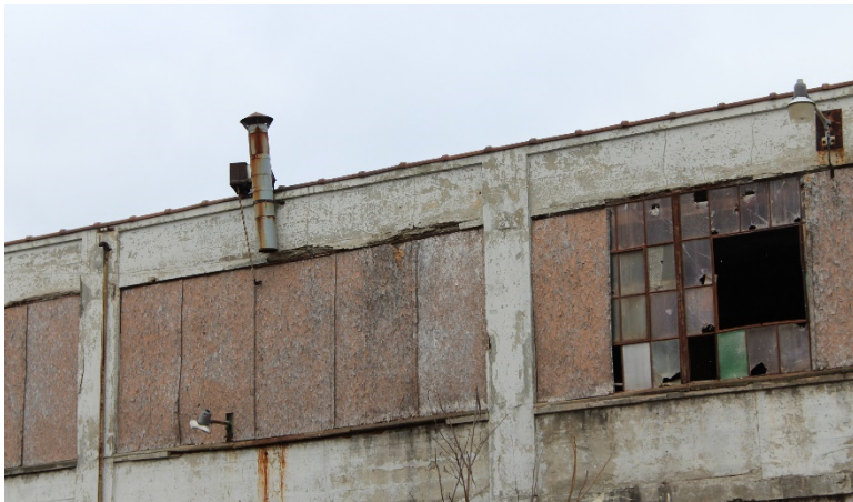
Photo 23 South Wall Area-D
